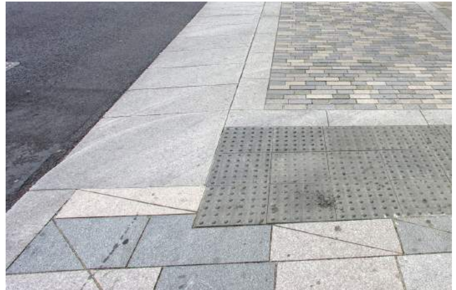
Elegant detailing of a continuous footway accommodating a vehicle change in level / Sidcup
