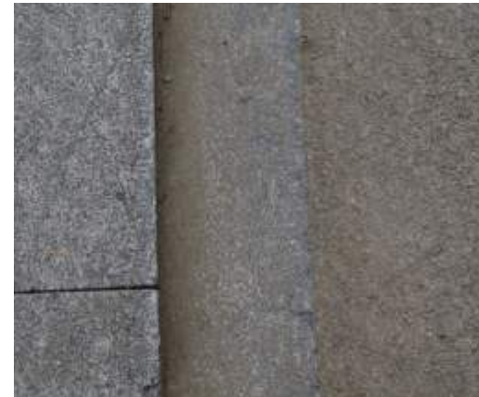
Granite kerb and granite kerb laid flat / form kerb zone. Example: Leyton High Road
