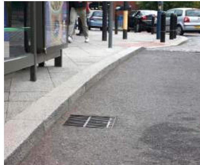
'Conservation' style kerb / natural stone aggregate in concrete kerb product, similar to various existing kerbs used in the town centre area. Example: St Albans
