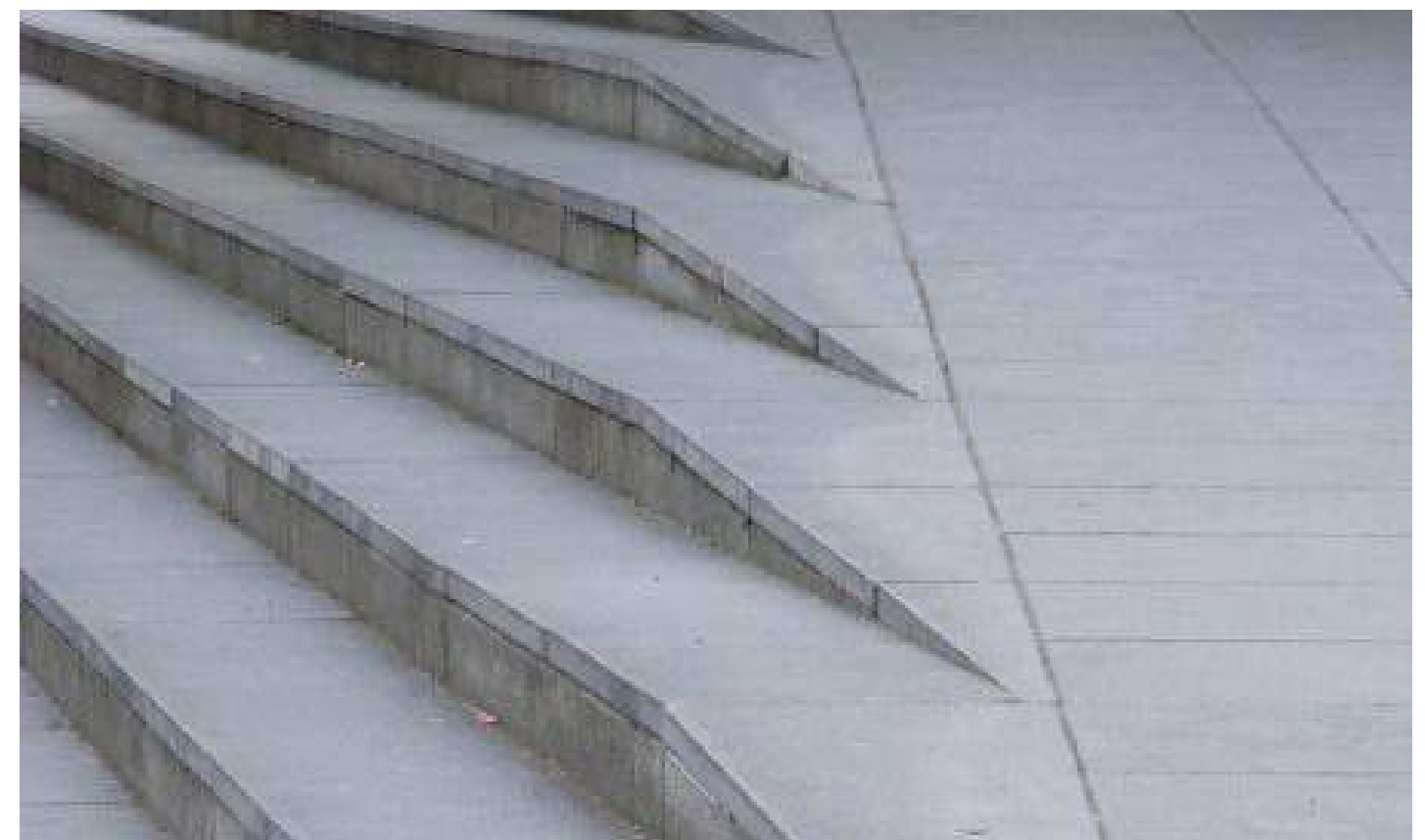
Steps and level changes need accurate and careful detailing / London
