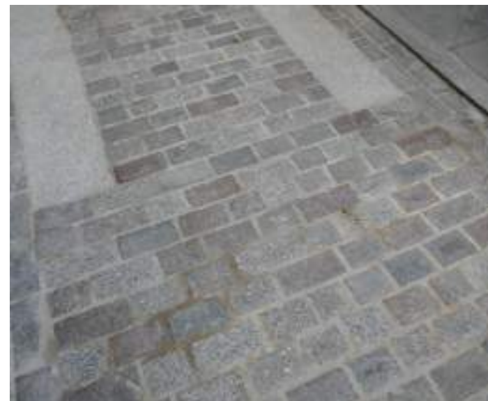
New laid kerbs / with two courses of setts laid longitudinally to form channels within the carriageway draining to traditional gully points in White Hart Yard, London
