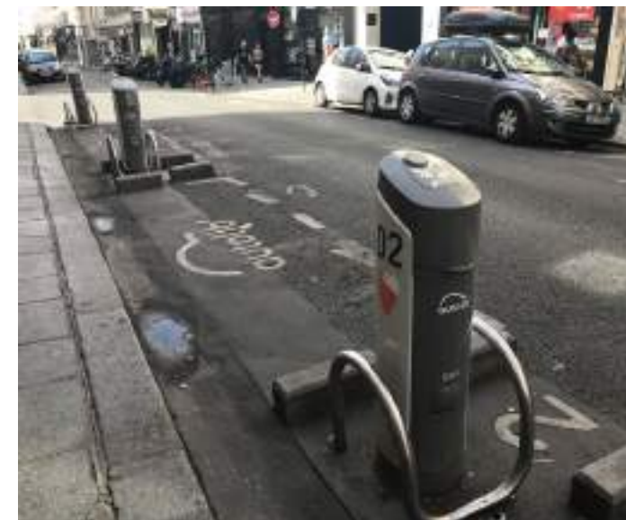
Efficient & unobtrusive charging banks / Paris
