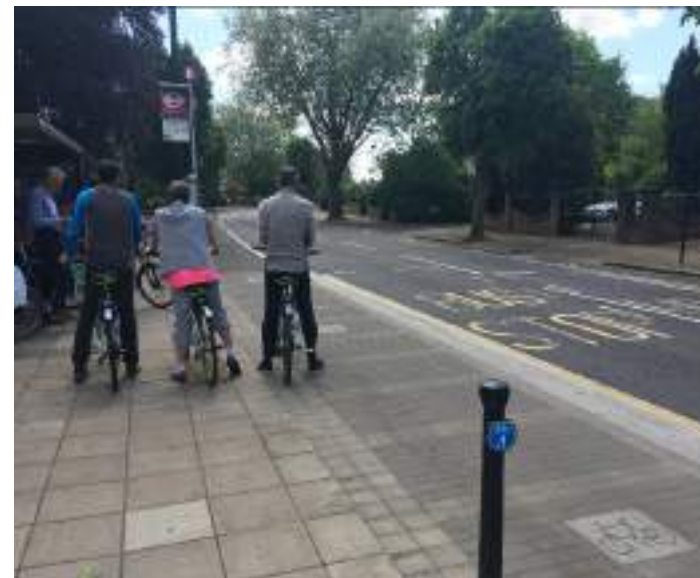
Block Paving / Used here on a bus border as a clear differentiation between footway and cycle track is made.
