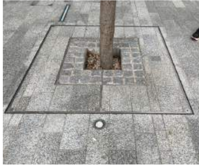
Typical coordinated and integrated heavy duty recessed tray / for newly planted trees in hardpaving ensuring flush natural stone finish with surrounding footways.
