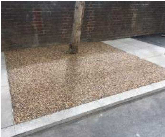
Resin bound gravel / finish to treepits where existing tree root protection areas are important in inner 'Town' areas.
