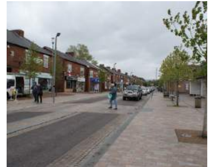
Extended kerbside channel / using 6 rows of small setts directs water flow and encourage responsible driving. In Poynton
