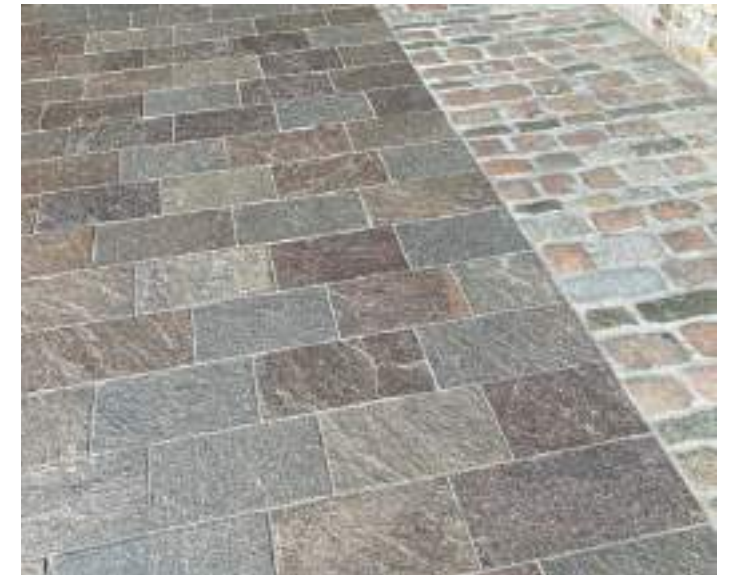
Porphyry flags / meet reclaimed granite setts at a building interface in Coal Drop Yards, London.
