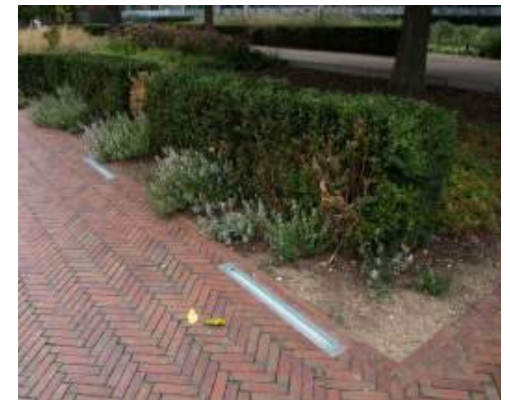
Clay Pavers and Edging to Public Footway / Moulded edge, 85mm wide x 200mm.
