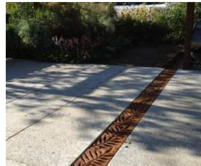
Decorative cast iron cover / channel drain cover in footway directing surface water to planted area. Iron Age Grates
