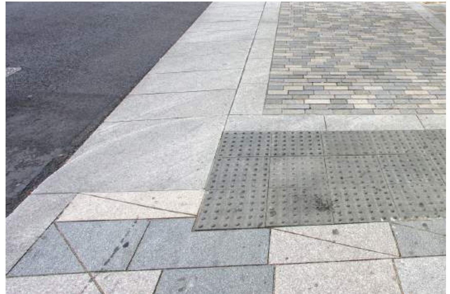
Good side street detailing / Sidcup
